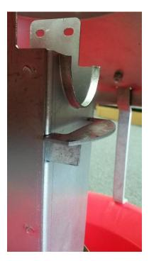
7. Place centering clip on feed line as shown below. Then snap on by firmly pressing on the clip. Note the orientation of the clip in relation to the tab on the feed line.
